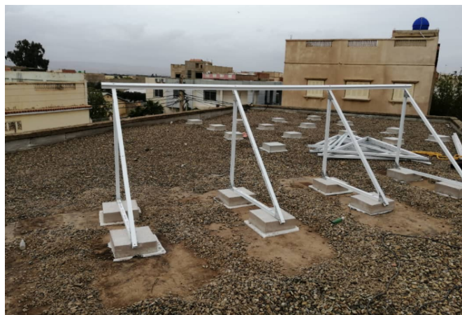
FIGURE 3.14 – Structure porteuse en aluminium.
