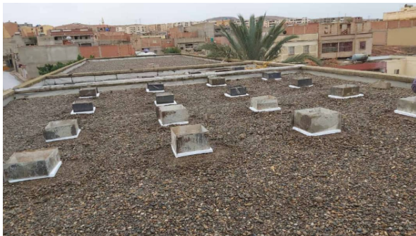
FIGURE 3.12 – Semelle de béton 50*50*20
