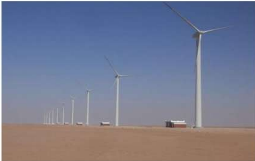
Figure 6: Wind power plant is located at Kabertene, Adrar
