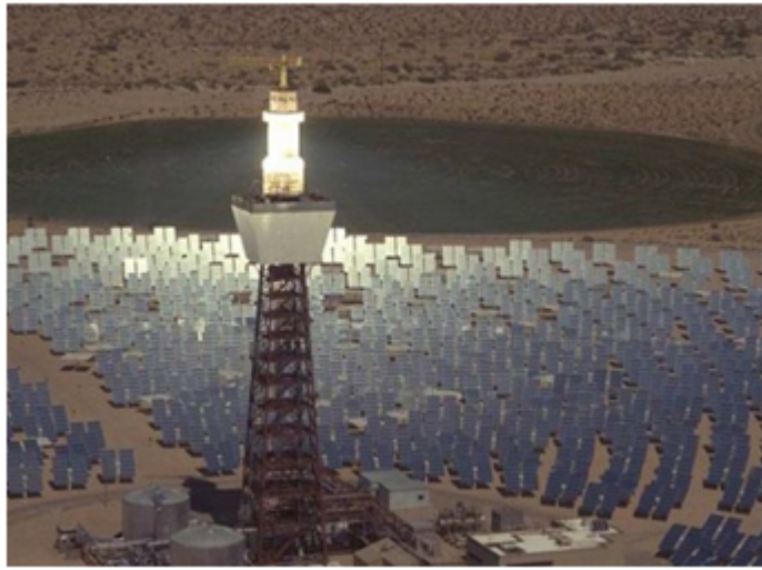
FIGURE 1.13 – Centrale photovoltaïque de Mojave, Californie (USA) [4].
