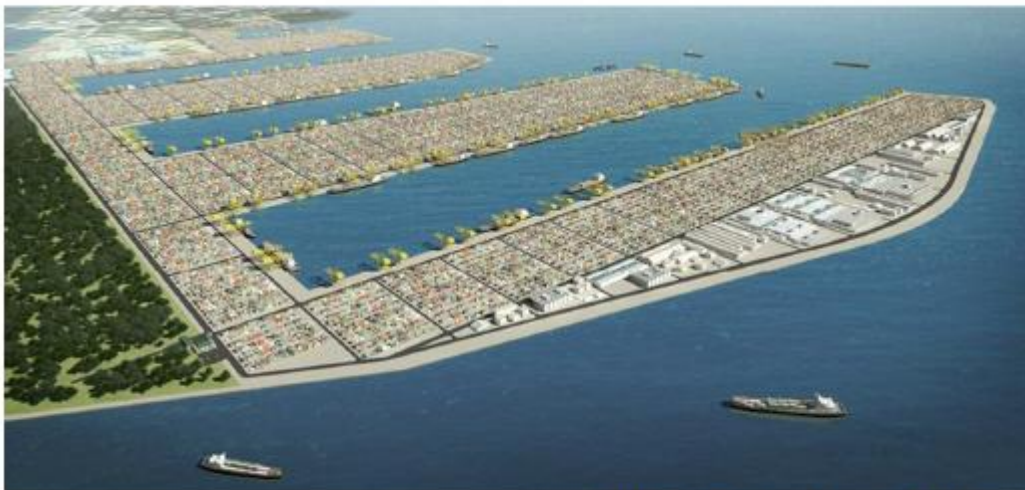
(b) Tuas Terminal in the Port of Singapore (Source: Maritime Singapore Connect, 2018 )
