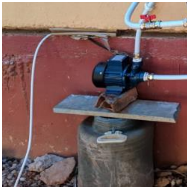
Figure III-15 Installation du moto-pompe.
