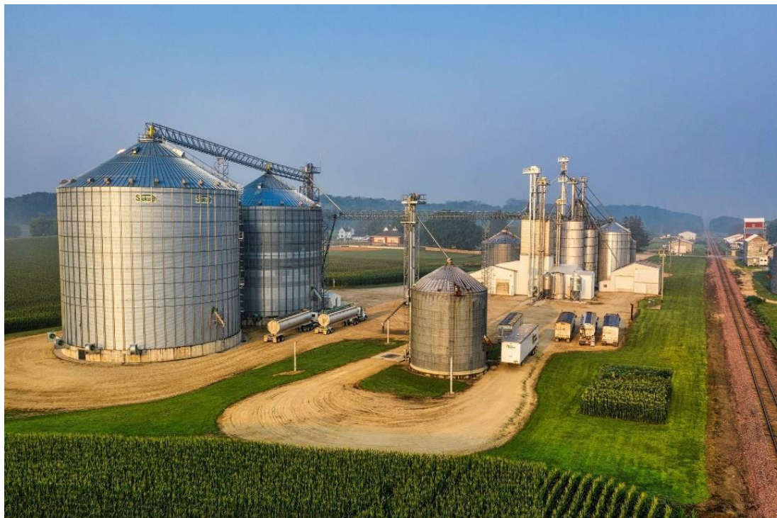
Figure 2.1: Silos de stockage [13]
