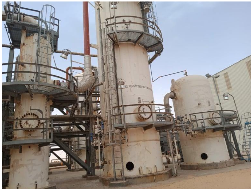
Fig 1.4: BP stabilization section [photo taken during the training]
