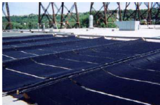
Figure 1.18: A Flat plate collectors without glazing [12]
